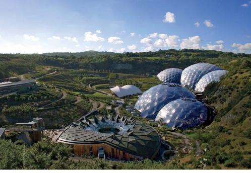
By developing a model based on bubbles, the team at Grimshaw solved the challenge of unpredictable ground levels for the Eden Project biomes
