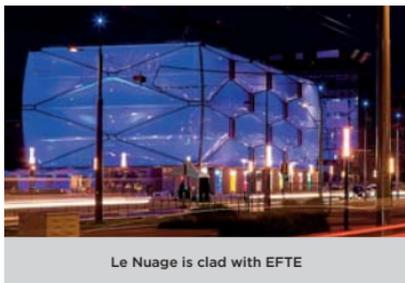
Le Nuage is clad with ETFE
