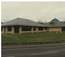
Refurbishment will transform the ageing facility
