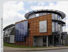
Modern PV panels can be installed on walls
