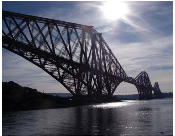
A visitor centre will be built into the base of the northern Fife tower
