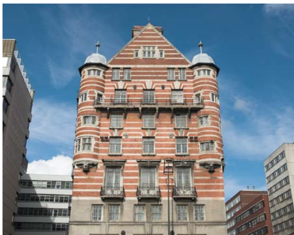
The portland brick Albion House is located on Liverpool's The Strand
