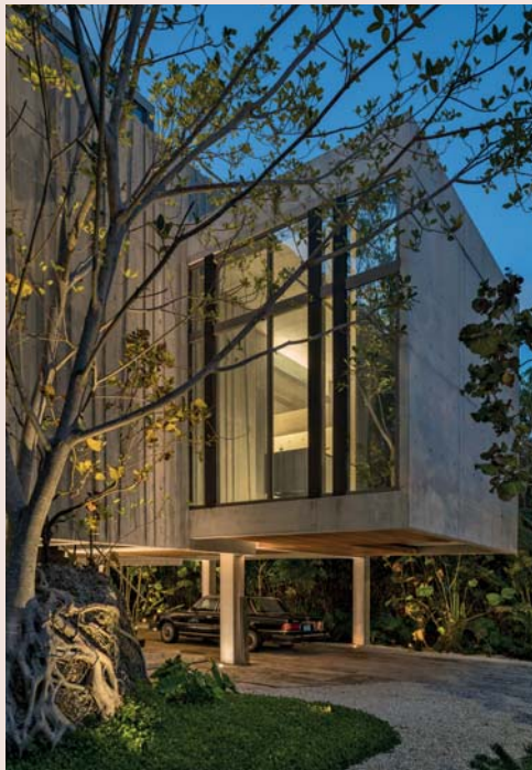
The raised design protects from flooding and allows air to circulate underneath
