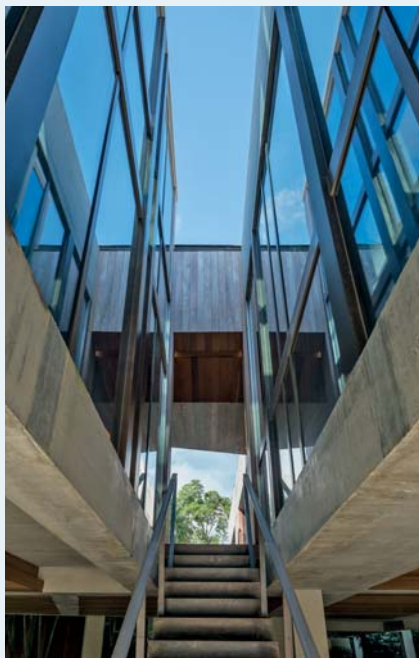
The retractable staircase lifts into the belly of the house when not in use
