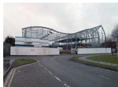
The centre's steel structure has been completed
