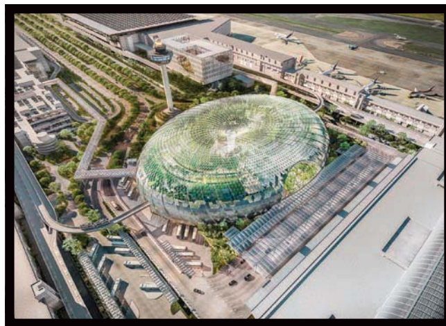
■ The dome will become one of the world's largest gridshells
