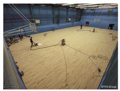
The new MVP floor is given a light sanding before the application of a Bona Supersport sealer.
