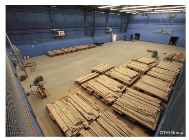
The substructure of the University's old court was refurbished before the new flooring could be laid.
