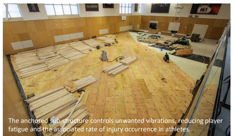
A self-levelling compound was applied prior to installing this highly engineered sub-structure.
